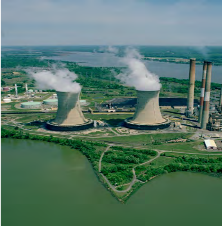
Exhibit 6-2. Natural draft cooling towers at Chalk Point Generating Station, Aquasco, MD
