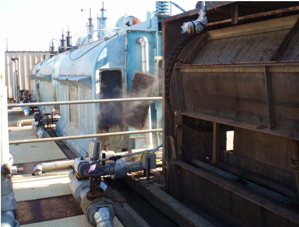
Exhibit 6-10. Traveling screen at Eddystone Generating Station, Eddystone, PA
